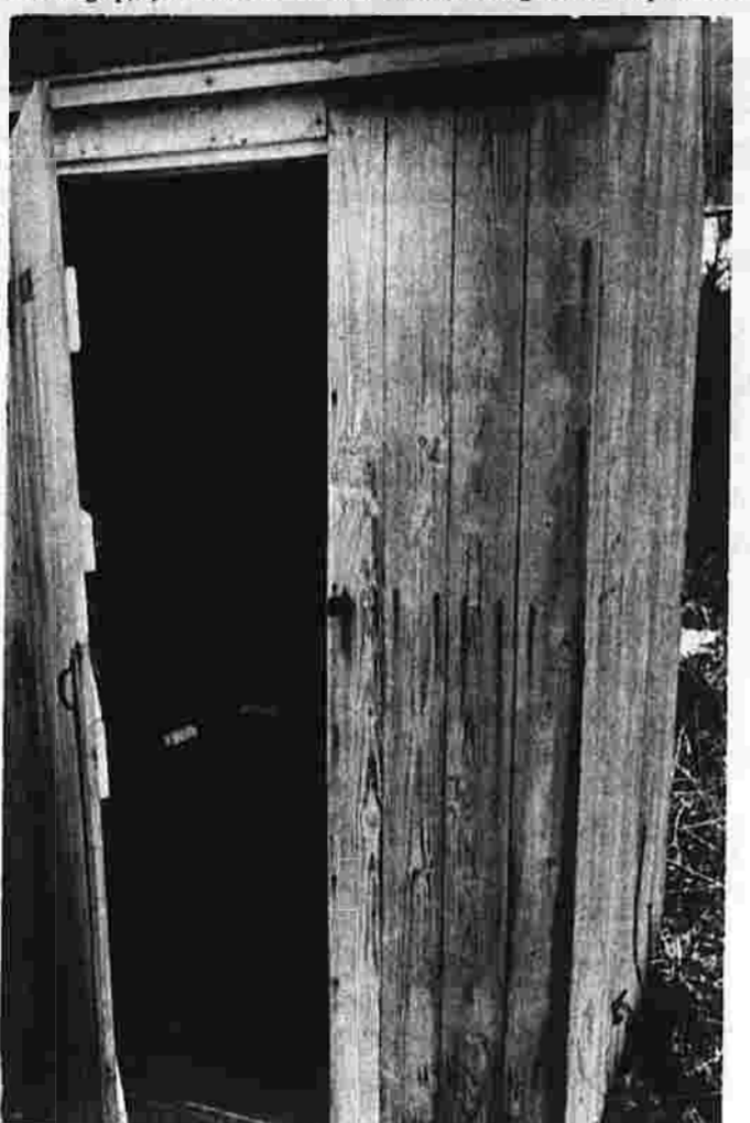
Early American This outshouse to the rear of the old Andover Town Hall is still in use. The hall does not have lavatories but is used regularly. (Herald photo by Dunn)
